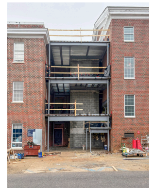
The new elevator tower.
